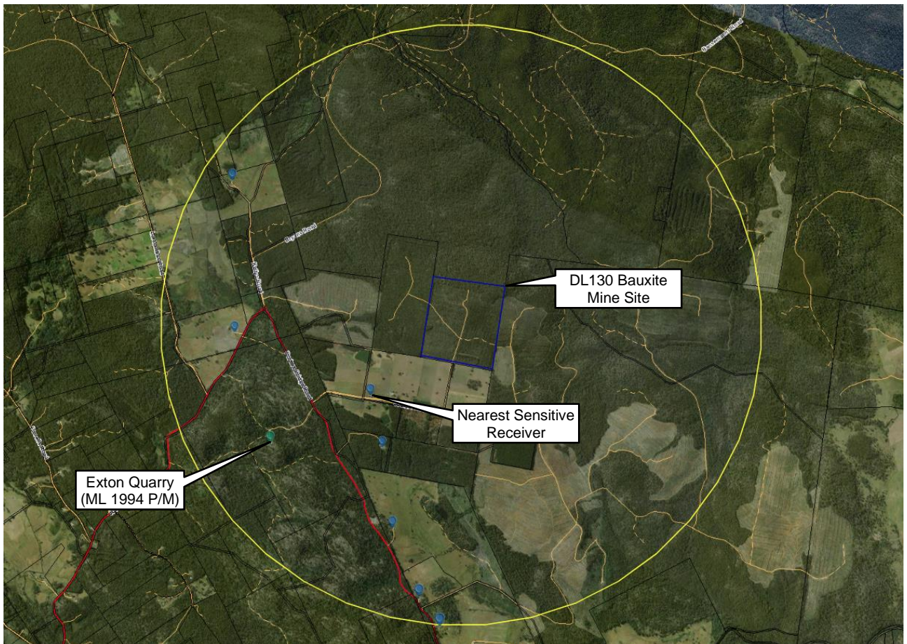
Figure 1: DL130 Bauxite Mine site (Blue) and surrounding area, including nearby residences (blue pins), existing major noise sources (green pins) and 3km radius (yellow). Basemap source: theList.
