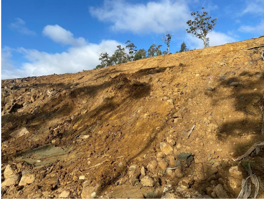
Figure 2 - landslide area reinstatement
