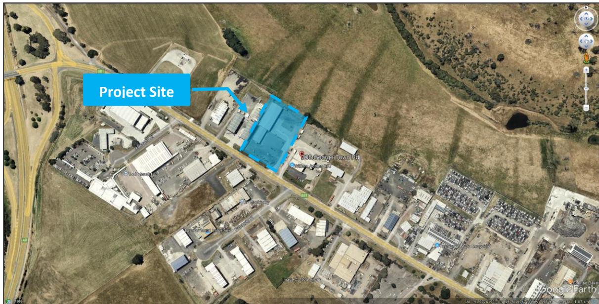
Figure 1 Location of Project Site (Image Source: Google Earth 2025)
