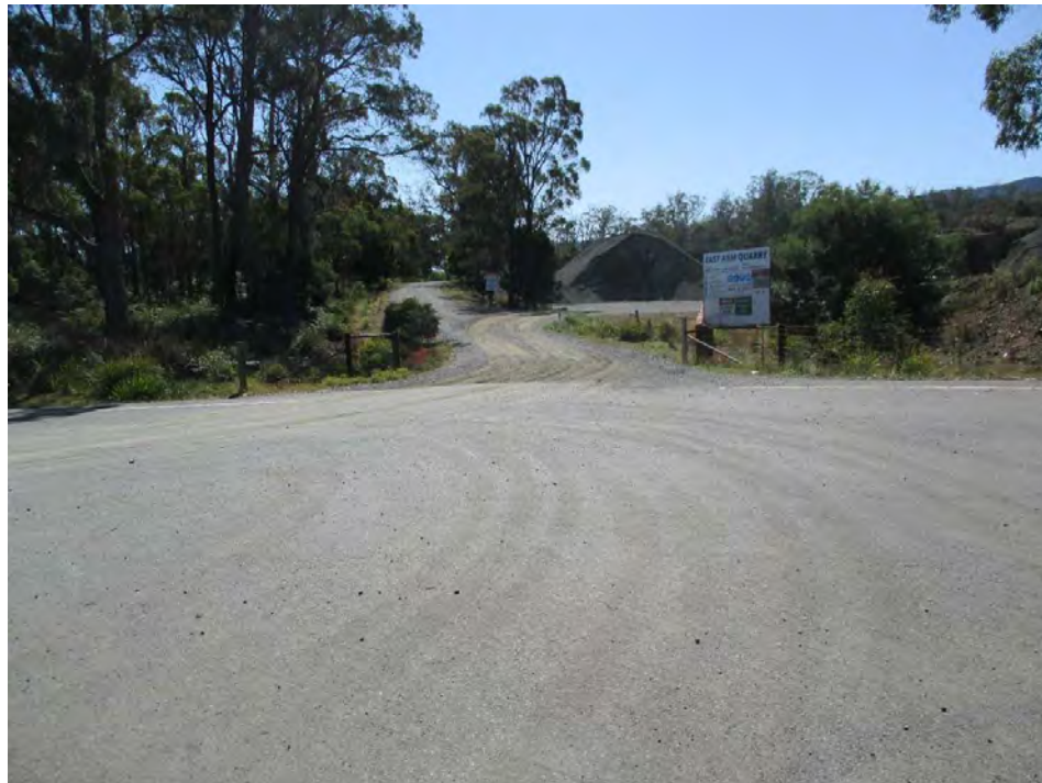
Photograph 3.1: View of access road to quarry site from East Arm Road
