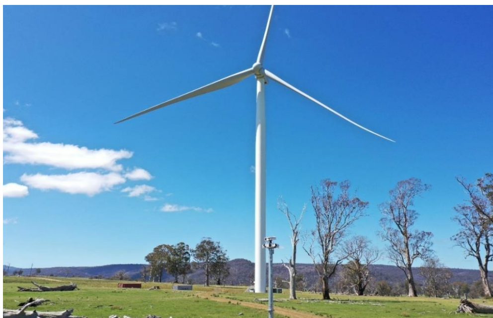
Figure 3-1: Cattle Hill Wind Farm showing GW140/3.0MW turbine and IdentiFlight station
