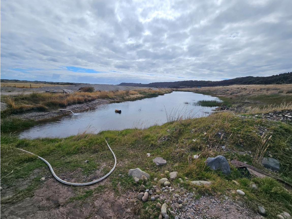
Process water dam (1 of 3)
