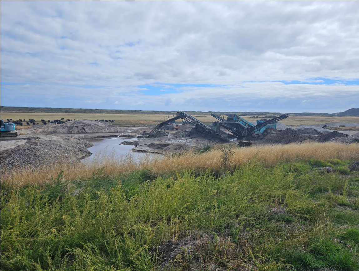
Screening process to settling pond No 1
