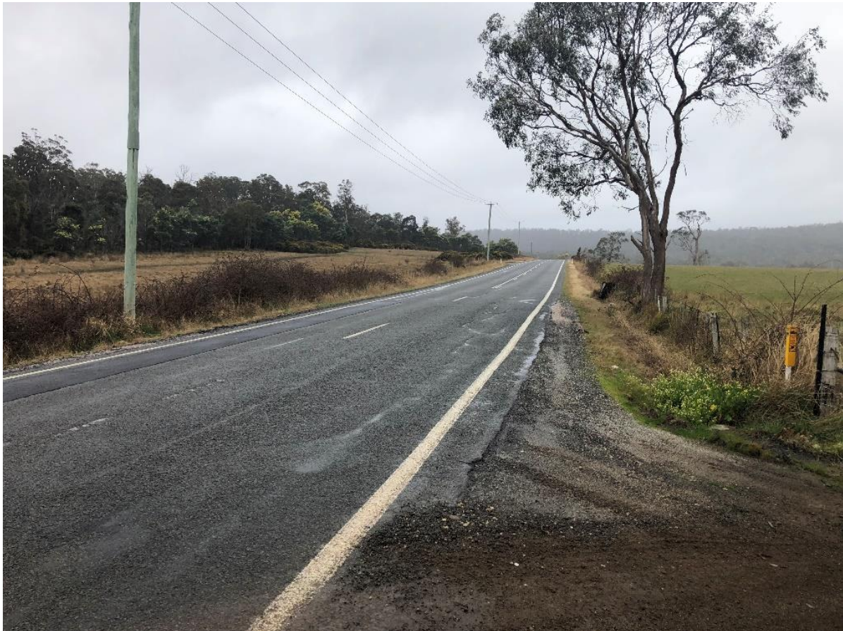
Figure 12. Line of sight on the Tasman Highway. North-east of the access point.
