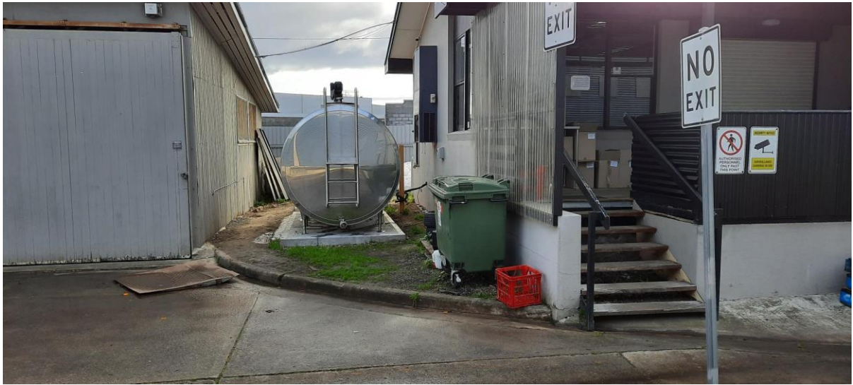
Image 1 – 56 Gormanston Road, Moonah Location of Vat Relative to Factory Building and Shed Building Location of Proposed Security Fence and Steel Upright Bollards
