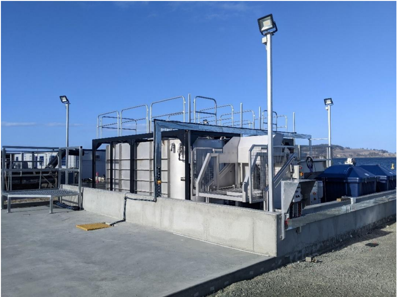
Figure 12 Electrona ensiling facility
