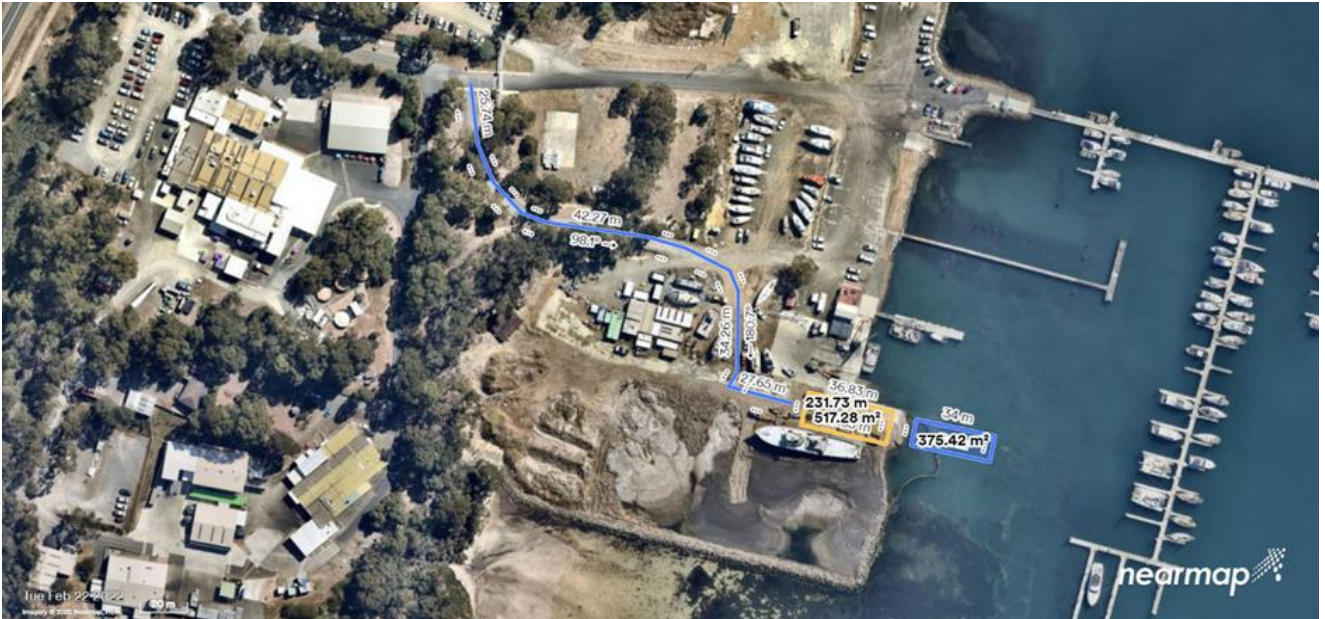
Figure 1 Primary loadout site at Margate Marina. Truck access (blue line) to rock stockpile (Yellow line) adjacent to the Curlew Vessel which is now land locked. The construction barge (blue rectangle) is in front of the rock stockpiling area.
