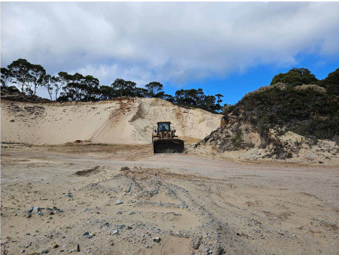
Existing excavation area – eastern boundary of lease
