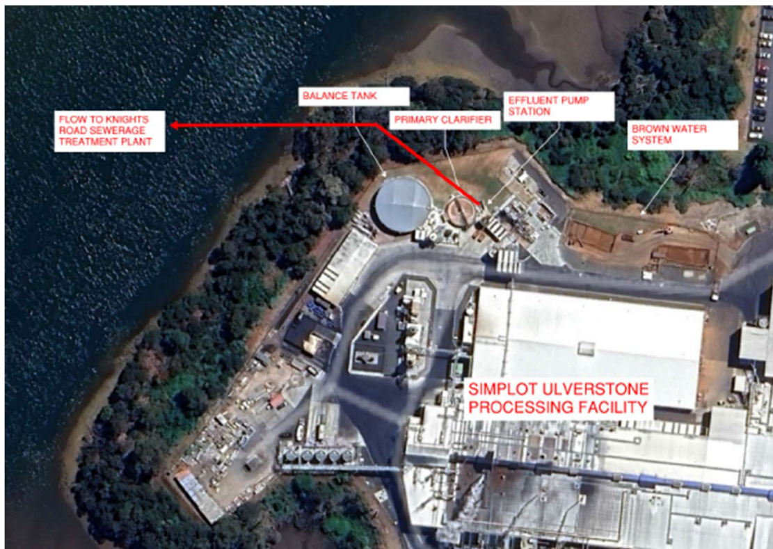
Figure 3 – Simplot Ulverstone Wastewater pretreatment system
