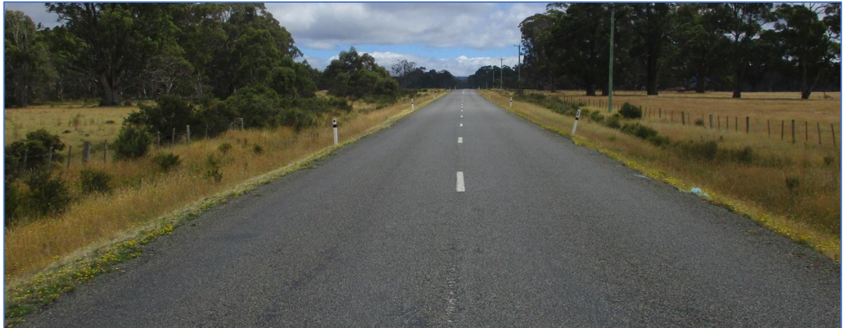
Photograph 9.3C- Available sight distance to the northwest (310 metres)
