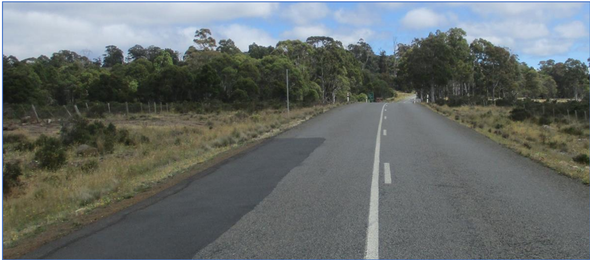
Photograph 9.4C – Available sight distance to the northwest (150 metres)
