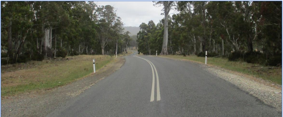
Photograph 9.1C – Available sight distance to the north (>500 metres)
