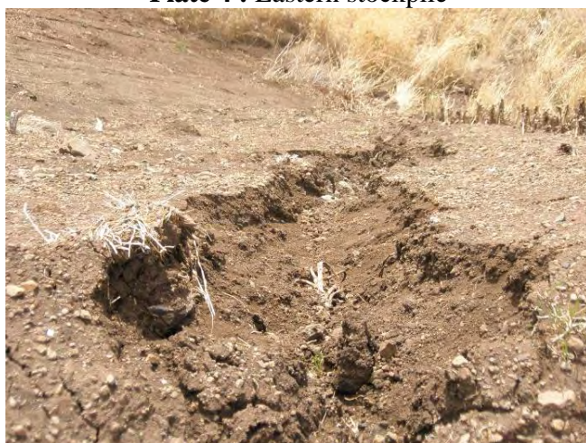
Plate 5: East facing batter erosion as a result of concentrated discharge
