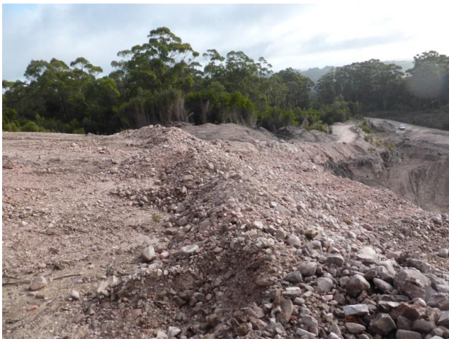
Figure 2. Overburden is well scalped back.
