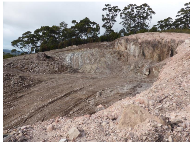
Figure 3. Active face and overburden.
