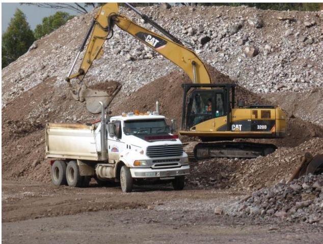
Figure 4. Material actively being removed.
