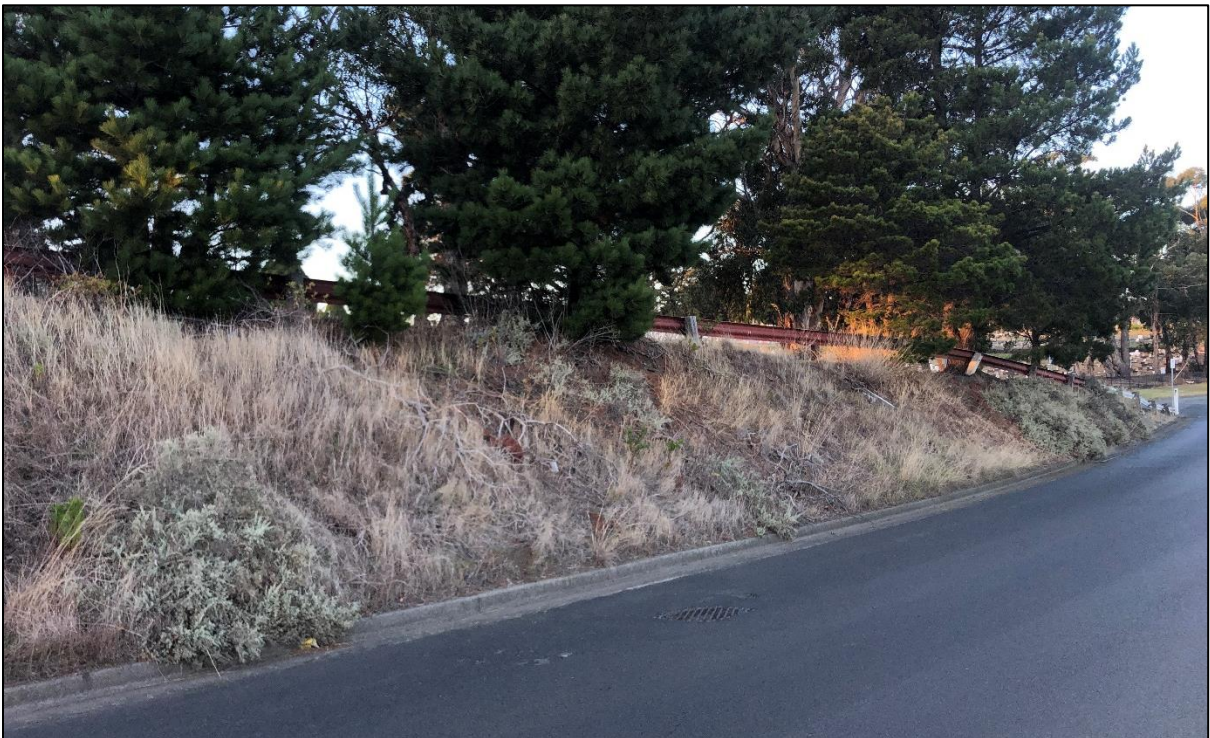
Plate 5. Typical composition of the road reserve in the project area.
