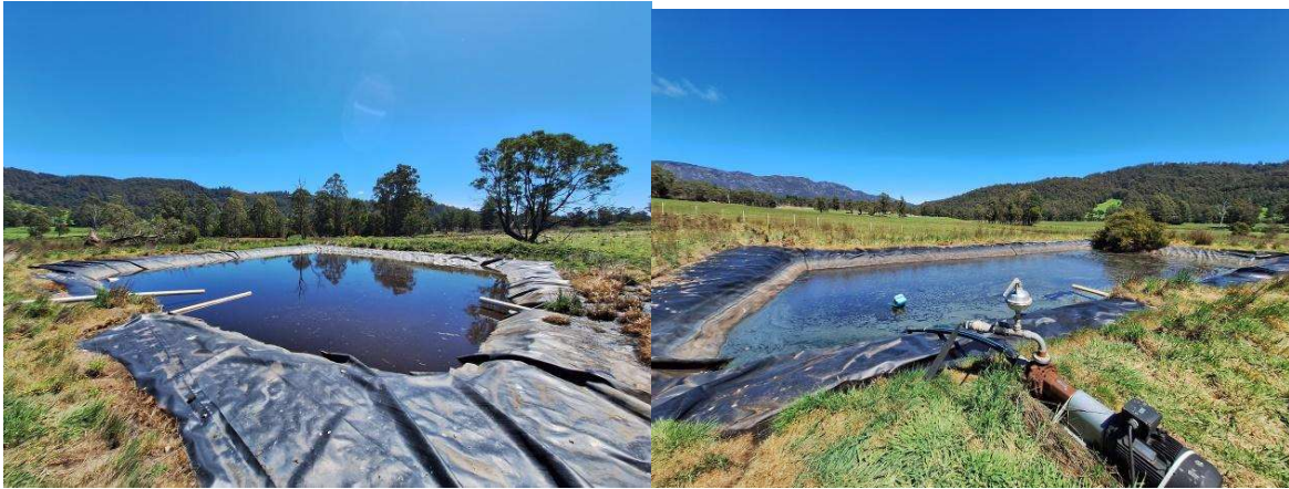
Figure 2 – Water Management On-Site (Primary Pond - First)
