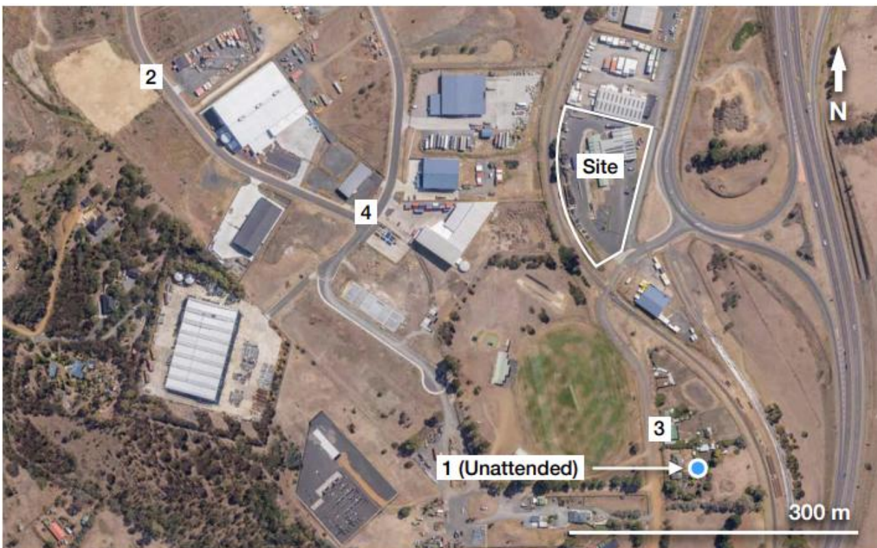
Figure 5: Noise monitoring locations (Figure 2.1 EER Appendix A).
